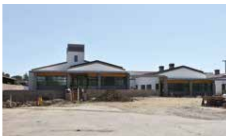
A recent snapshot of construction and progress, May 3, 2019.
